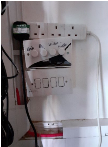
Photographs above show a broken light switch, burnt socket and gland covers missing on a distribution board.
