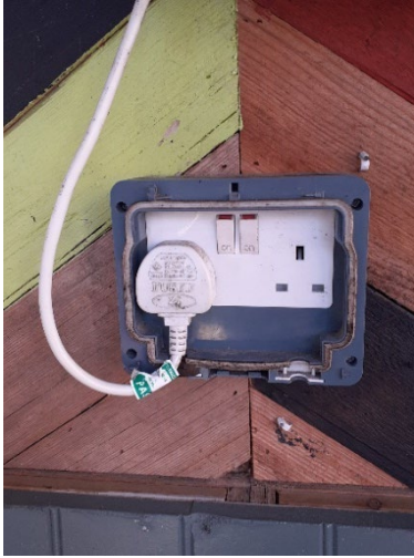
Photographs above show an outdoor socket with cover missing, live cables and missing switch covers exposing live cables.
