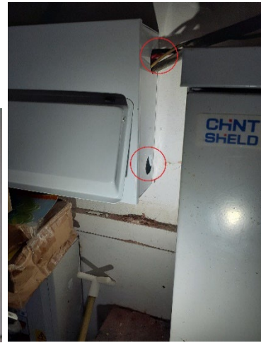
Photographs above show a broken light switch, burnt socket and gland covers missing on a distribution board.
