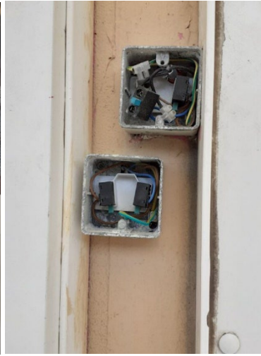
Photographs above show an outdoor socket with cover missing, live cables and missing switch covers exposing live cables.
