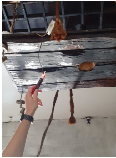
Photographs above show an outdoor socket with cover missing, live cables and missing switch covers exposing live cables.
