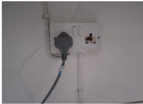
Photographs above show a broken light switch, burnt socket and gland covers missing on a distribution board.
