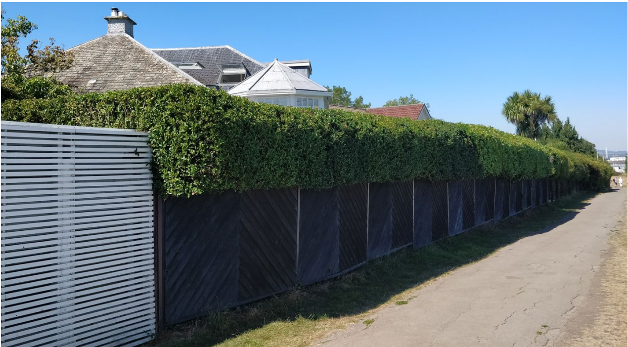
Rear elevations of dwellings back onto Cliff Walk
