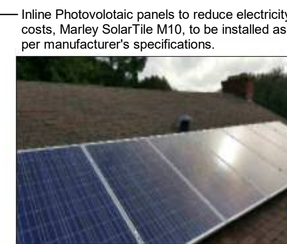
Inline Photovoltaic panels to reduce electricity costs, Marley Solar Tile M10, to be installed as per manufacturer's specifications.
