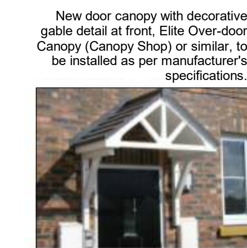
New door canopy with decorative gable detail at front, Elite Over-door Canopy (Canopy Shop) or similar, to be installed as per manufacturer's specifications.
