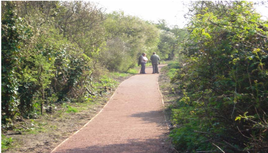
(Completed footpath improvement works)
