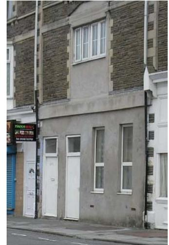
*The above properties have been poorly converted to residential uses, with little regard to replicating the proportions and architectural detailing found on the first and second floors and the use of non-matching materials.*
