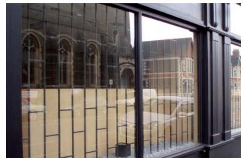
External security shutters that are substantially perforated, slotted or the lattice type may be considered acceptable, provided they meet the following criteria:
