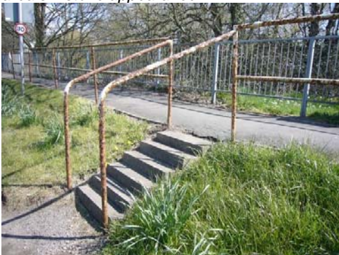
Railings to the footbridge across the River Ely are in need of enhancement.
