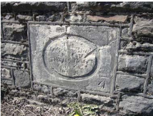
Eroded plaque on the side of the river bridge. The bridge is a locally listed County Treasure.
