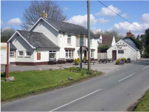
In common with most buildings in the area, The Sportsman's Rest has a slate roof.
