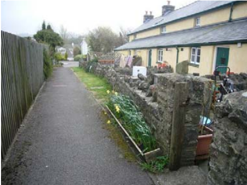
A stonewall forms the boundary of Church Row's small rear gardens.
