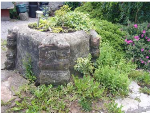
The wellhead is in need of attention.
