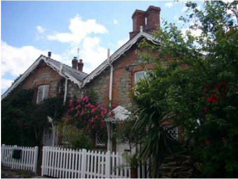
Nos 1, 2 and 3 Church Cottages.
