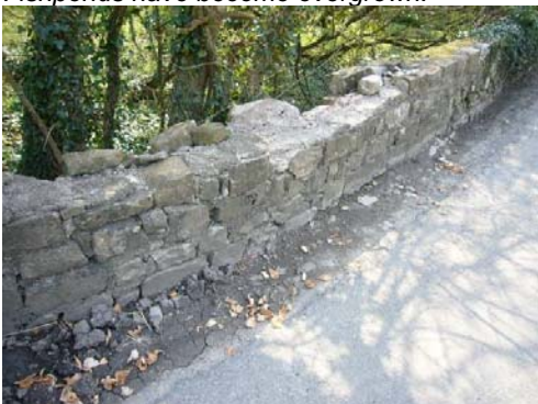
The parapet of the road bridge is in need of repair.
