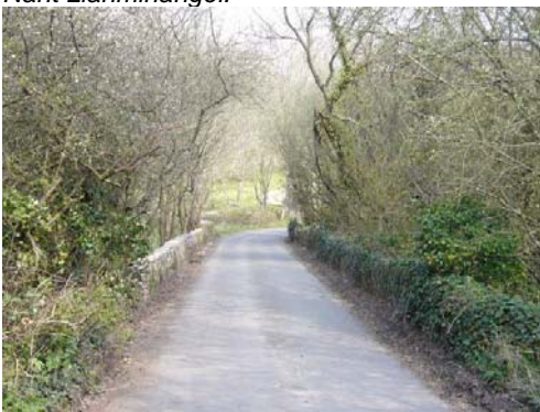
An 18 th century stone road bridge crosses Nant Llanmihangel.
