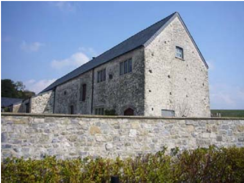
The 17 th Century stone barn, beside the manor house, is now converted to residential use.
