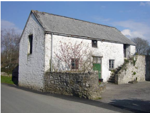
Barn to the East of Great House
