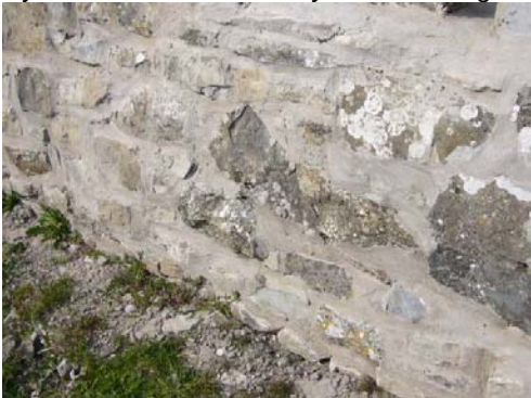
Incorrectly pointed stone work can spoil the appearance of a wall.
