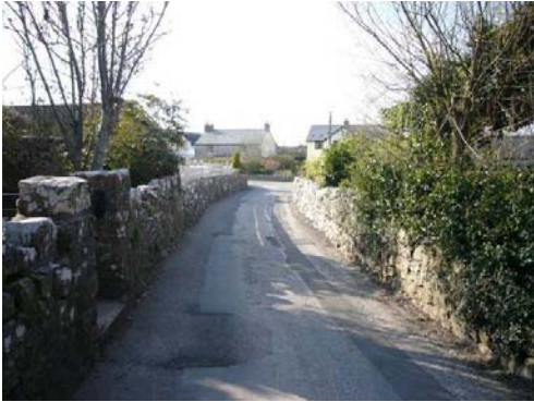
Roadside stone boundary walls are a prominent feature of the area.
