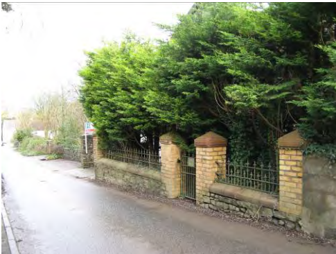
Original railings and gate remain at New House.
