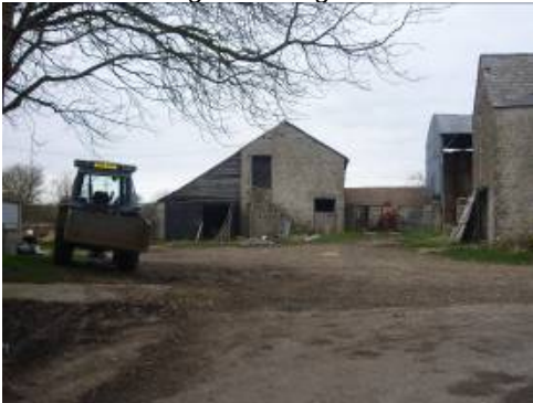
The farmyard at Llancadle Farm is one of the most significant open spaces in the conservation area.
