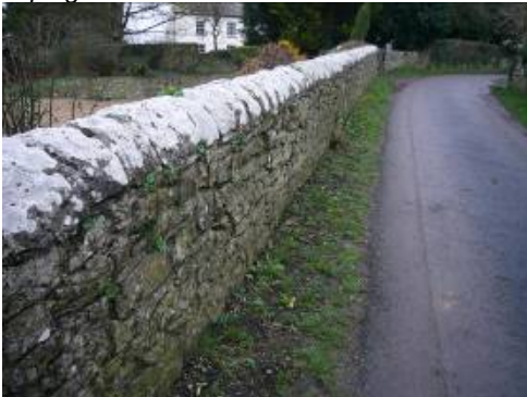
Stone wall with half-round coping stones.
