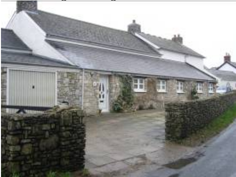
Lower Llancadle Farm, stone-built but much altered and bounded by a traditional stone wall.
