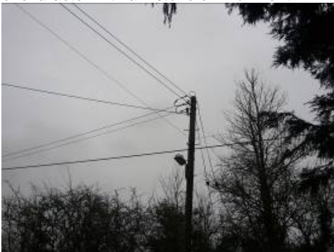
Wires and cables intrude upon the streetscene.
