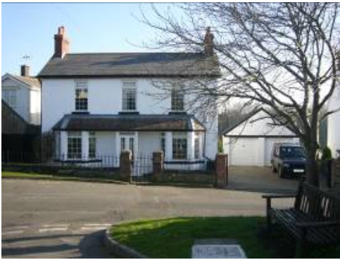
Penybryn and The Manse (opposite) are late 19th century buildings that add to the area's historic interest.
