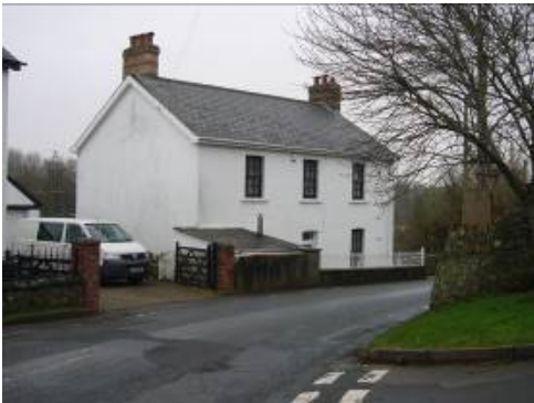
The Manse stands below the level of the road accentuating the village's hillside location.
