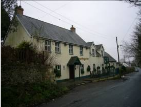
The Green Dragon was formerly thatched but has been rebuilt after being damaged in a fire.
