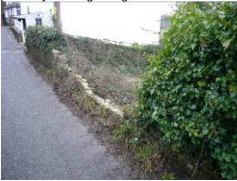
Part of the stone wall beside The Manse has collapsed and is in need of reconstruction. The adjoining field is in poor condition.
