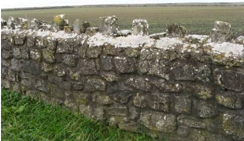
Detail of local limestone wall.
