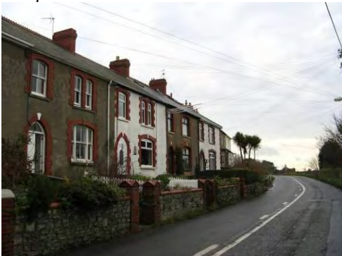
There is no pavement outside Station Terrace.
