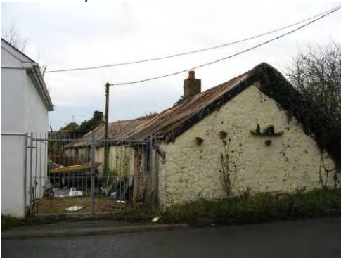
Outbuilding next to the Bethel Baptist Chapel is in poor condition.
