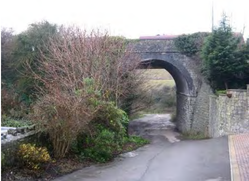
View down Well Road towards the railway bridge.
