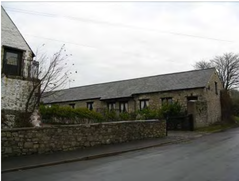
A number of former barns have been converted into residential use.
