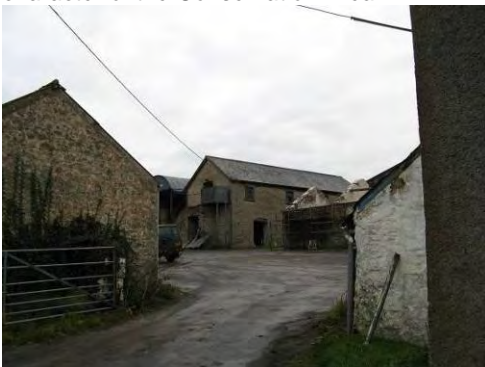
Barns at Upper House Farm, some of which are in disrepair.
