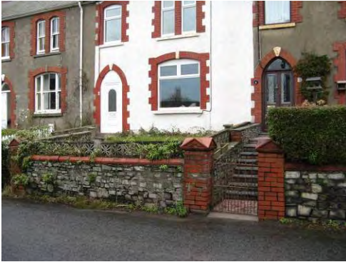
Details of stone wall at Station Terrace.
