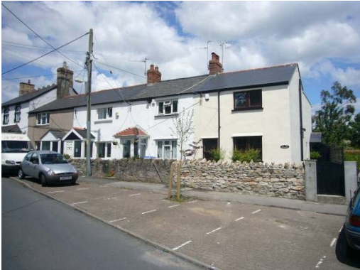
This row of houses, built c.1850, has been much altered and lost much of its historic interest.
