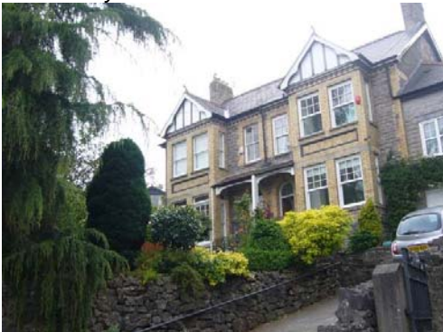
A pair of large semi-detached dwellings built soon after the arrival of the Barry railway.
