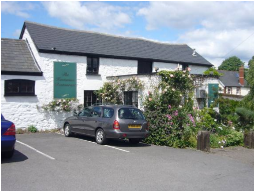
Barn at rear of Star Public House
