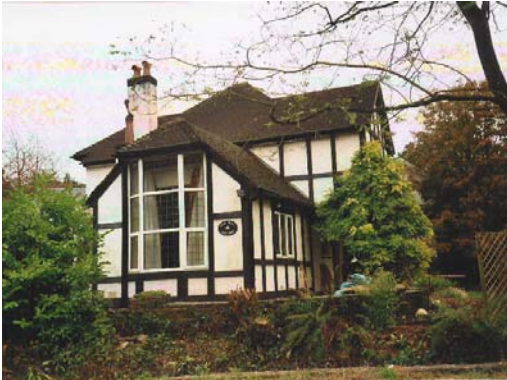
Mill House, Mill Road
