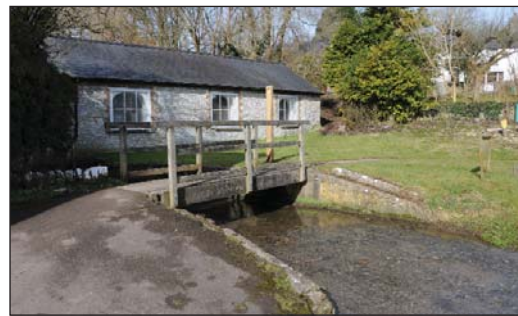
The former woollen mill and footbridge/ford at Factory Road.
