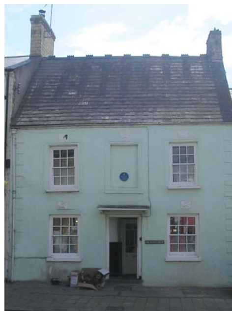
The Ancient Druid, Eastgate: a house of mediæval origins but now of 18th C external appearance, characteristic of the 'layering' of historic periods to buildings in Cowbridge.
