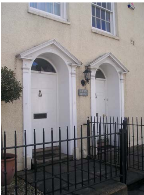
Nos. 56 and 58, Eastgate: a pair of late Georgian houses with much original detailing and forecourt enclosed by railings.
