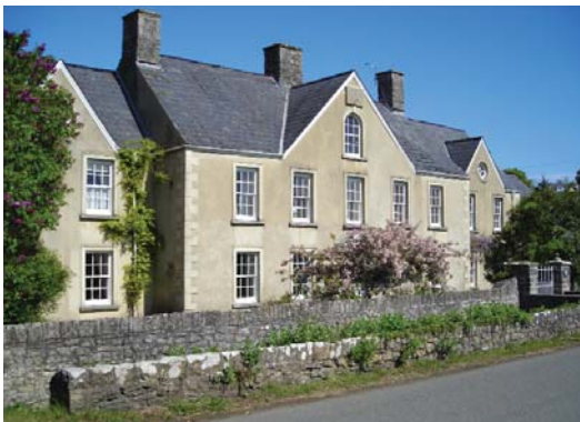
Great House: a highly listed early Georgian house.
