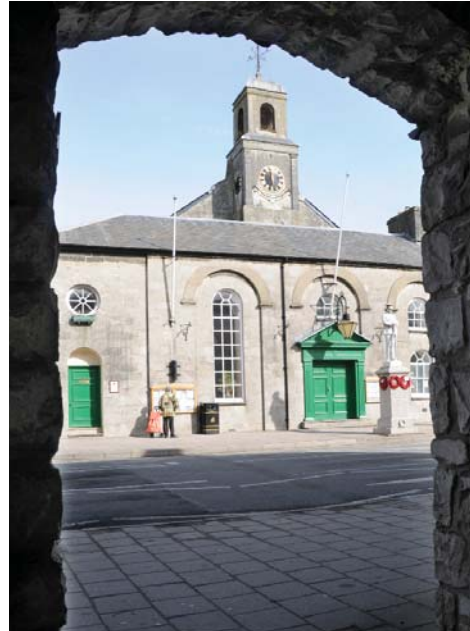
Cowbridge Town Hall: a fine late Georgian public building with landmark tower, bellcote and cupola.
