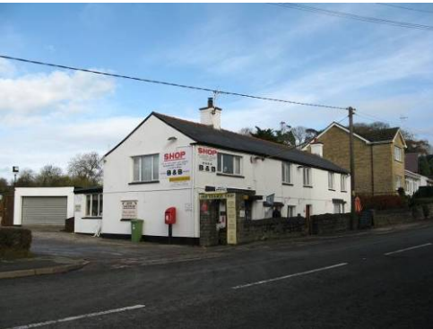
Cluttered signage to the Village Shop.
