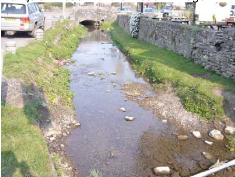
The stream widens before flowing through a culvert under the main road.
