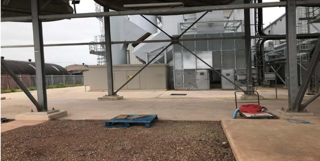
31. This structure is also located on the north-east elevation and the rectangular structure with double doors shown centrally within the above photograph. The developer has confirmed the dimensions as 600 L x 220 W x 290 H (area 13.2 sqm) and that the structure was installed on 01.02.2018 and houses valve sets necessary to distribute fire water to the deluge system.
