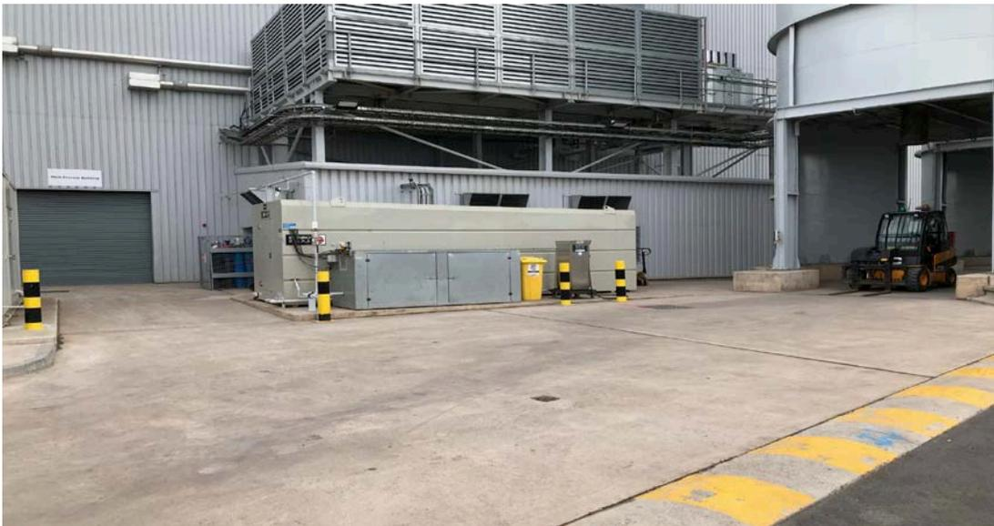
21. This structure is also located on the north-east elevation located centrally within the site and within the centre of the above photograph. The developer has confirmed the dimensions as 12508 L x 7350 W x 4231 H or 9754 if auxilliary coolers are included (area 27.5 sqm). It was installed on 01.09.2017 and the structure houses air compressors that can no longer fit in the main building.
