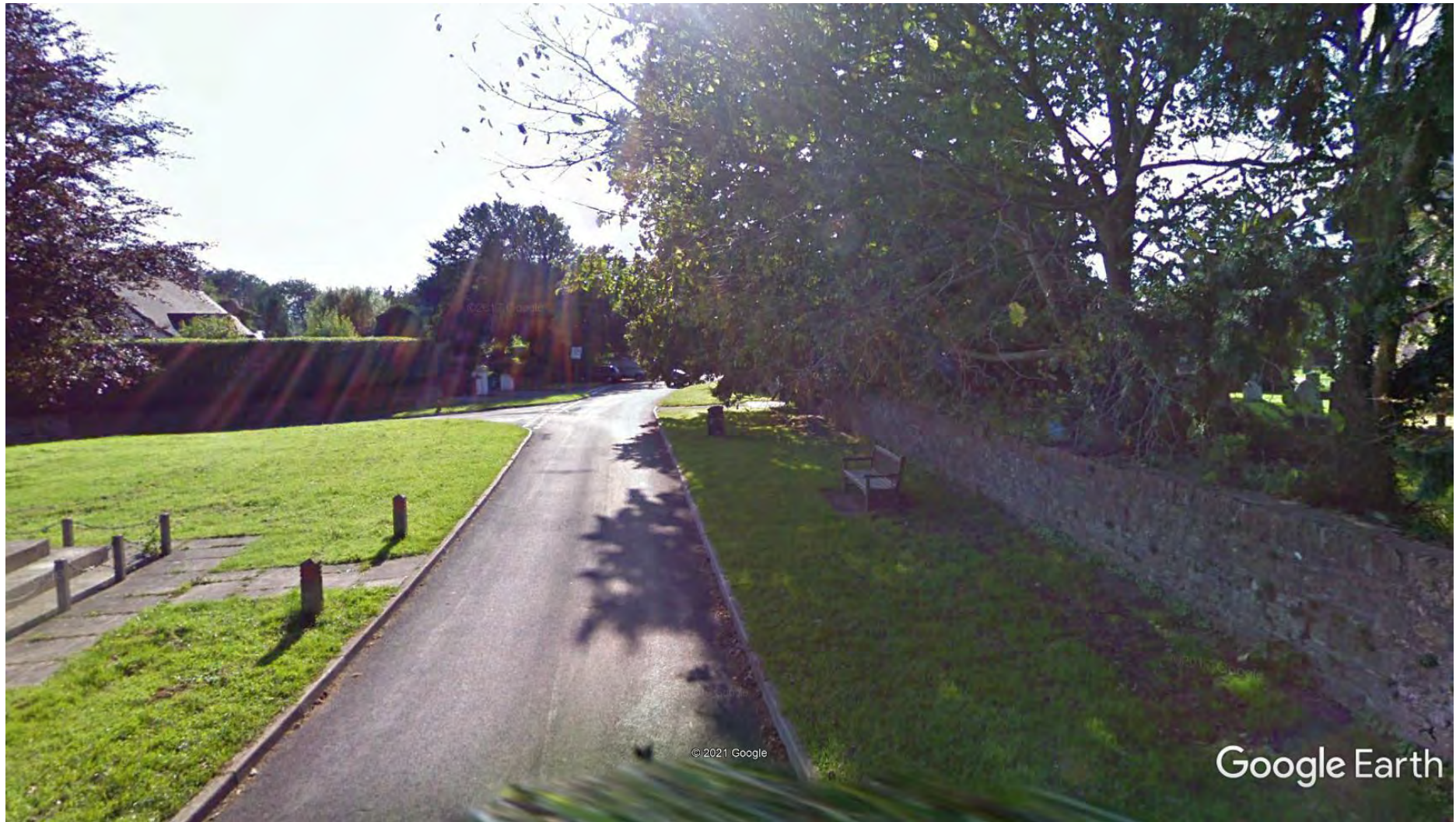
8. School Lane southern side of Church
