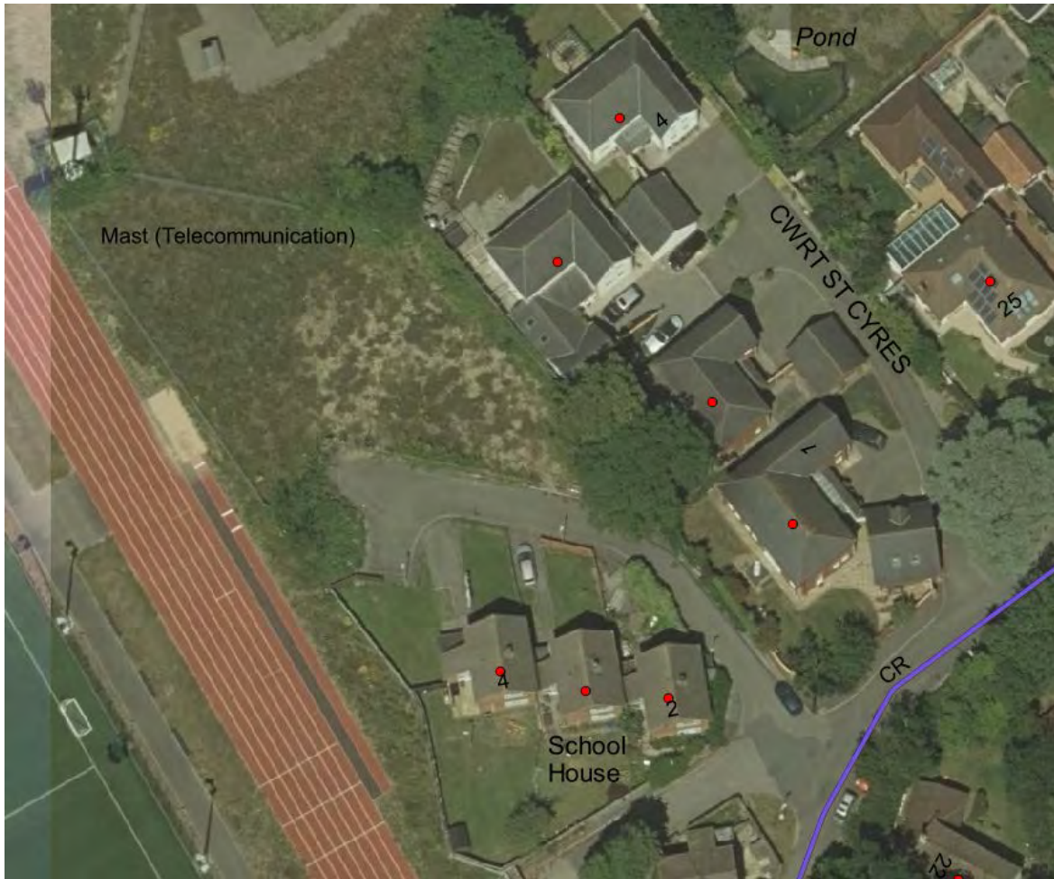
Photograph 5 – Aerial photograph (2017) showing position of site relative to neighbouring properties, to St Cyres Road (indicated by purple line) and St Cyres School running track to the west
