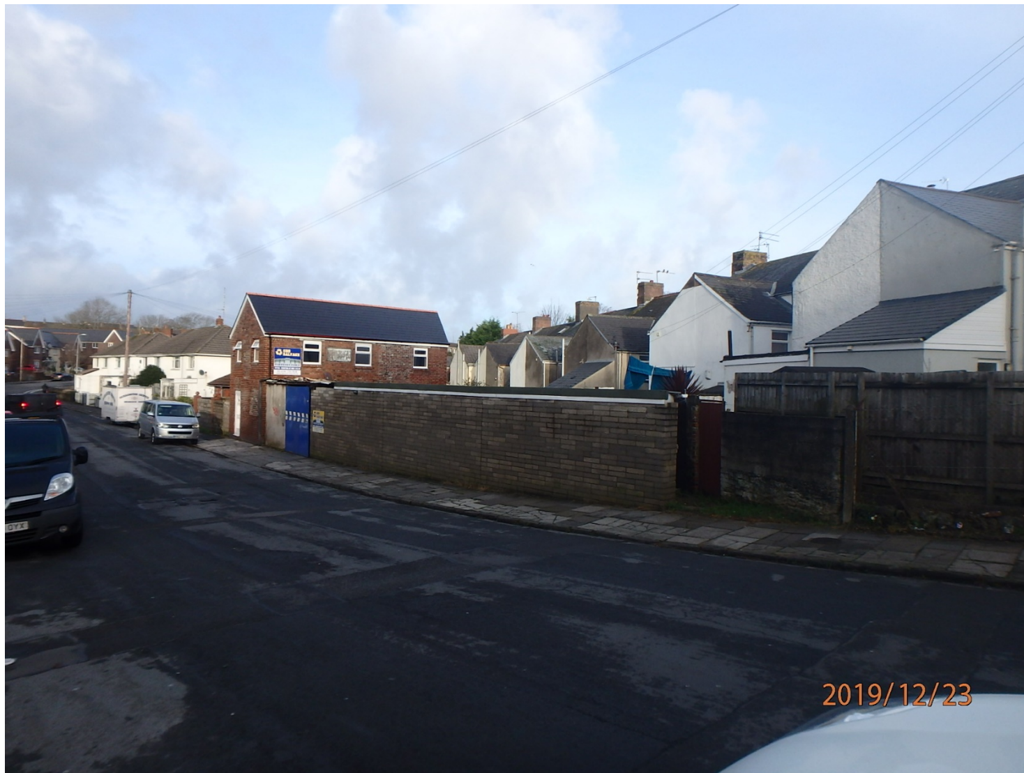
Site photograph 1 - The building prior to commencement of works
