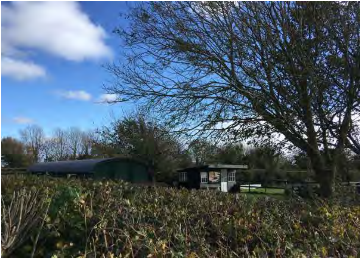
VIEW OF RAILWAY LUGGAGE VAN BODY AND STATION BUILDING FROM ADOPTED HIGHWAY
