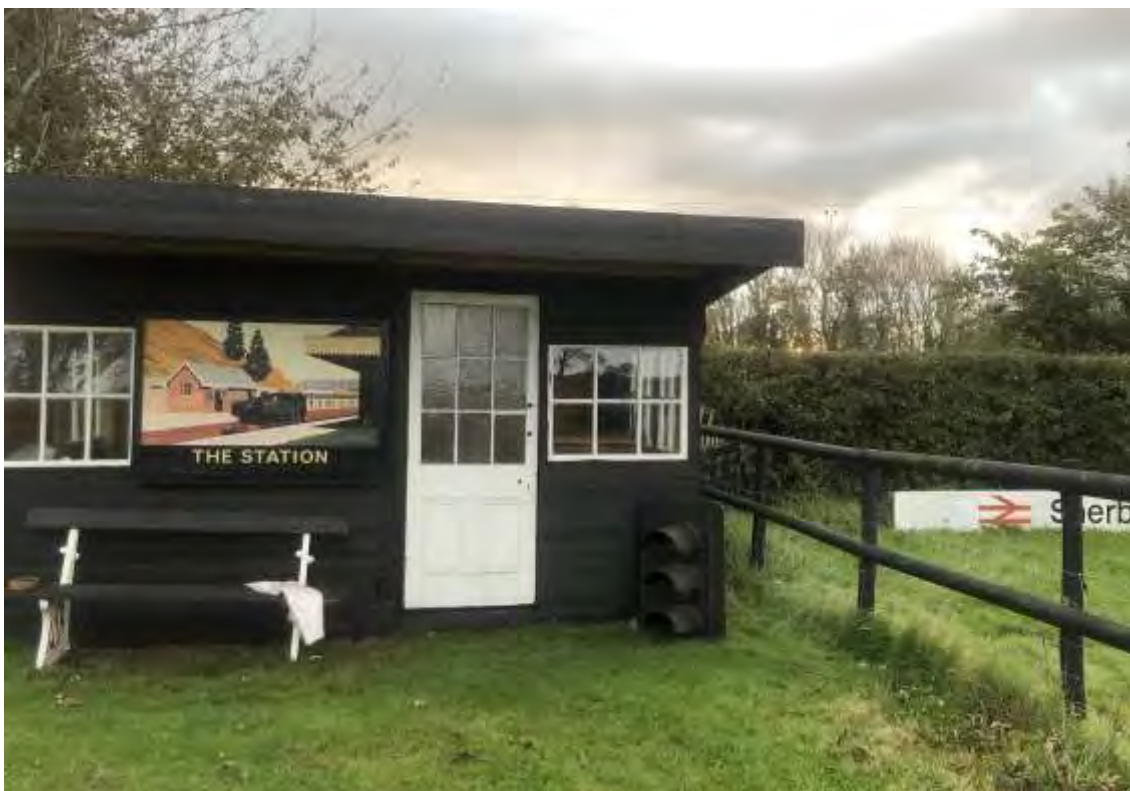
VIEW OF STATION BUILDING FROM WITHIN THE SITE
