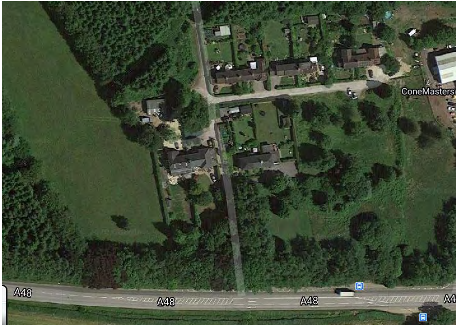
Aerial view of the site and surroundings
