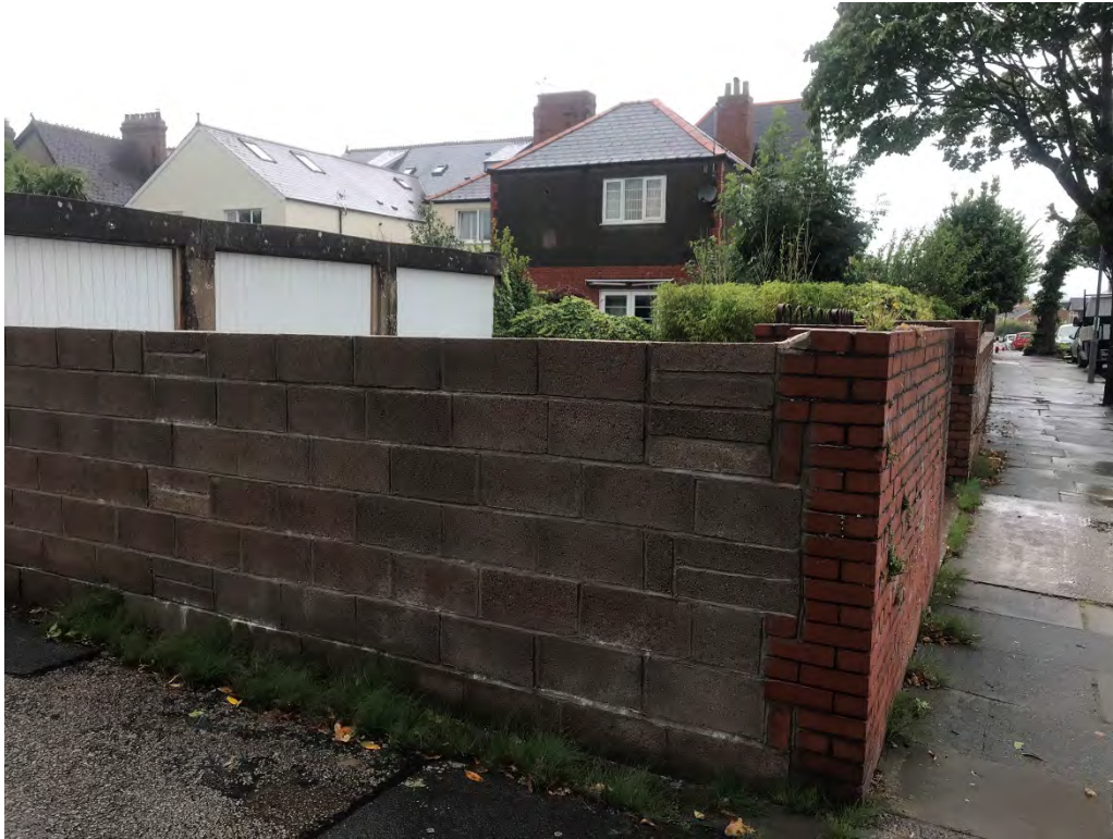
View into the site from Roseberry Place showing the wall fronting rear service lane and rear of properties along Stanwell Road.
