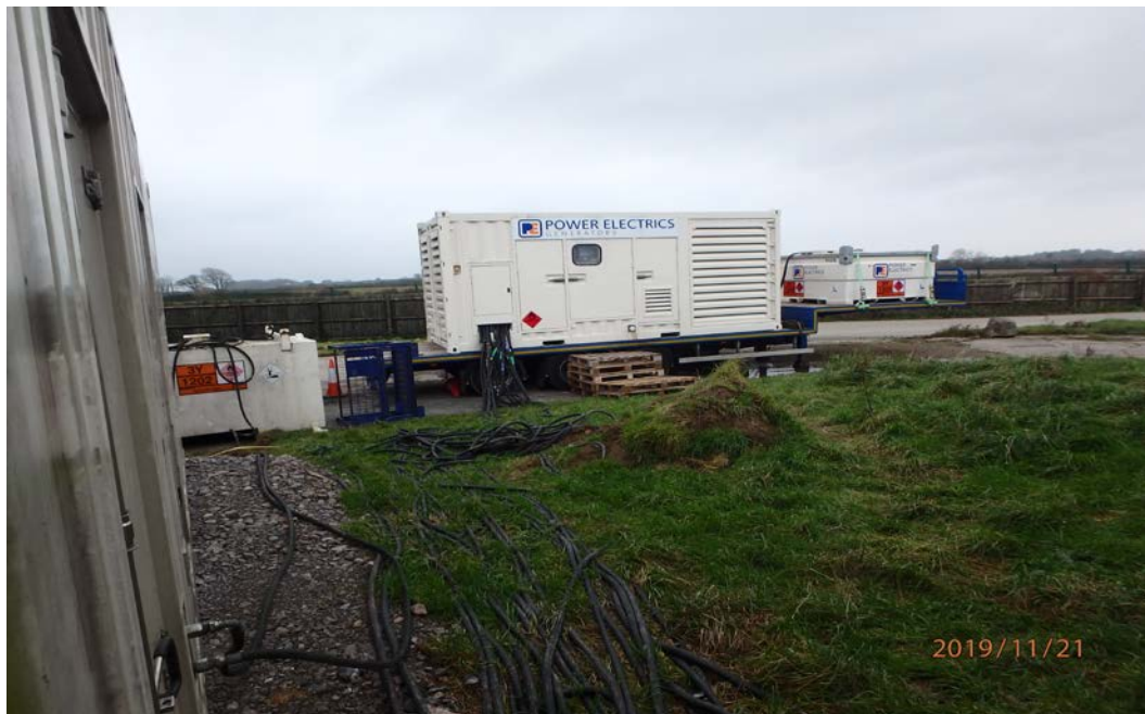
Photo 3. - temporary operational generator - located to south-west of Hangar A.
