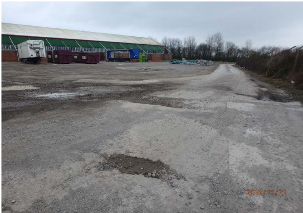
Photo 2. - existing northern boundary and haul road.
